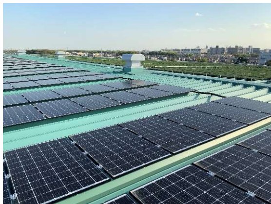
MT Tokyo Metropolitan Distribution Center
