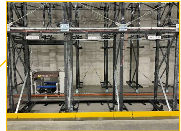
● Ready-to-pick warehousing system
